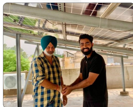
Pakhawal Road Ldh. – 10 kW (WAAREE)
