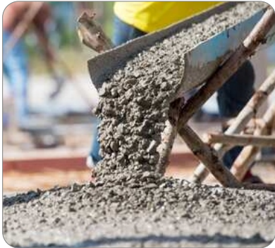
Civil Work & Installation Material
